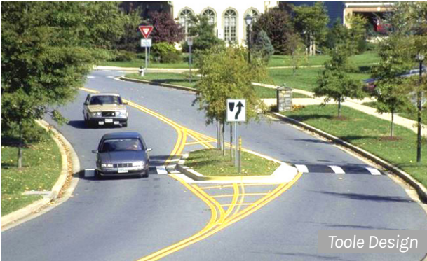
Speed humps installed on hills help slow traffic coming downhill
