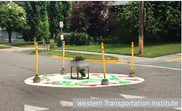
Traffic Circles can be quickly and cheaply installed as Pilot Projects
