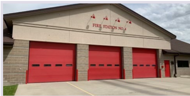
Old asphalt shingle roof with EIFS Siding
