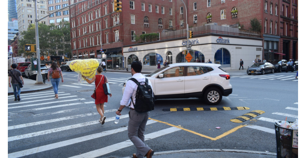
Temporary turn wedges can be installed to test turning radii
