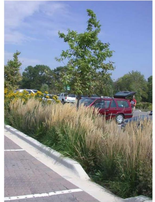
Fig. 27-1200.G: Curb cut to allow drainage
