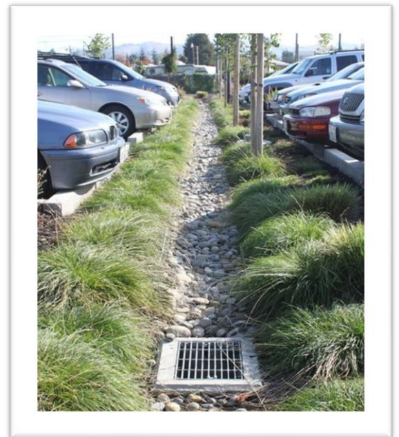
Fig. 27-1200.E Left: Landscape islands with storm water infiltration.
