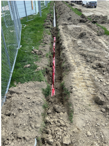
New 6" Irrigation Line and Electrical Conduits w/ tracer tape
