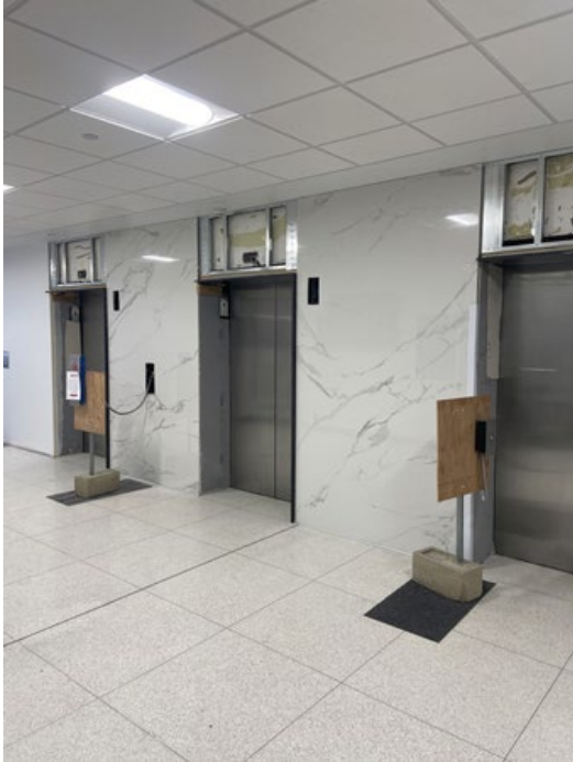
4 th Floor Install large format tile on elevator wall.
