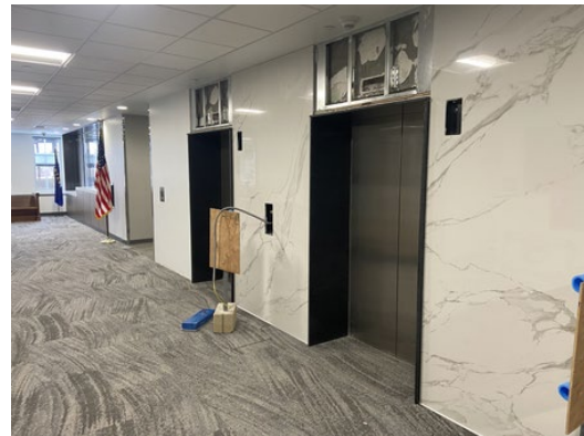
2 nd Floor Install large format tile on elevator wall. Install blocking for roller shade in room 245.
