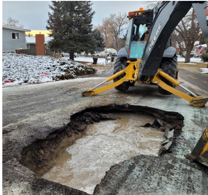
Fairway Drive Water Main Repair Jan 2024
