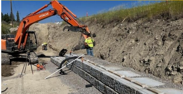
Building Retaining Wall @ Skyline Trail
