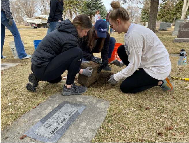
Volunteers replace a headstone after leveling and bringing the headstone back to grade
