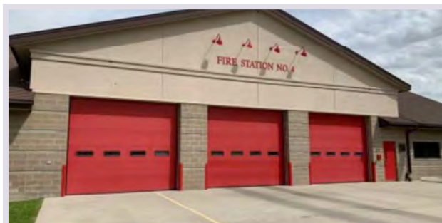
Old asphalt shingle roof with EIFS Siding
