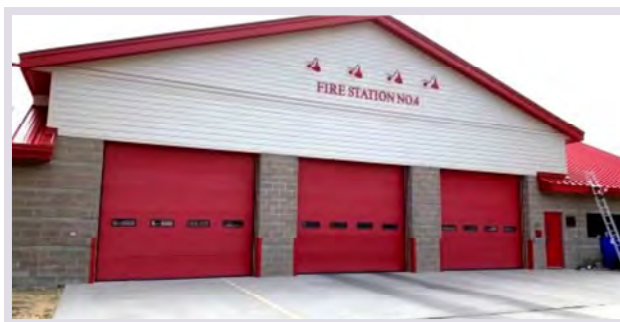
New metal roof and cement board lap siding
